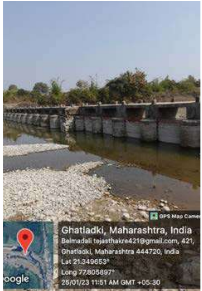
GP : Ghat Ladki Structure: Check Dam
