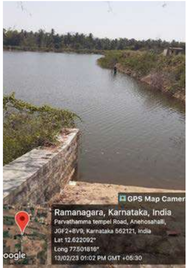
GP : Ramnagara Structure : Farm Pond
