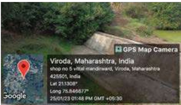
GP : Viroda Structure: Gully Plug/Nala Bund
