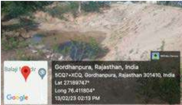
GP : Tilwar Structure : Percolation Pond
