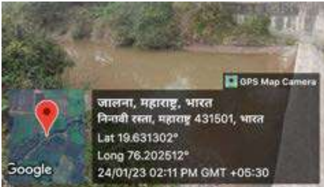
GP : Amba Structure: Drainage Line Treatment
