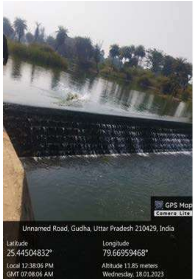
GP- Thathewara Structure- Percolation Pond
